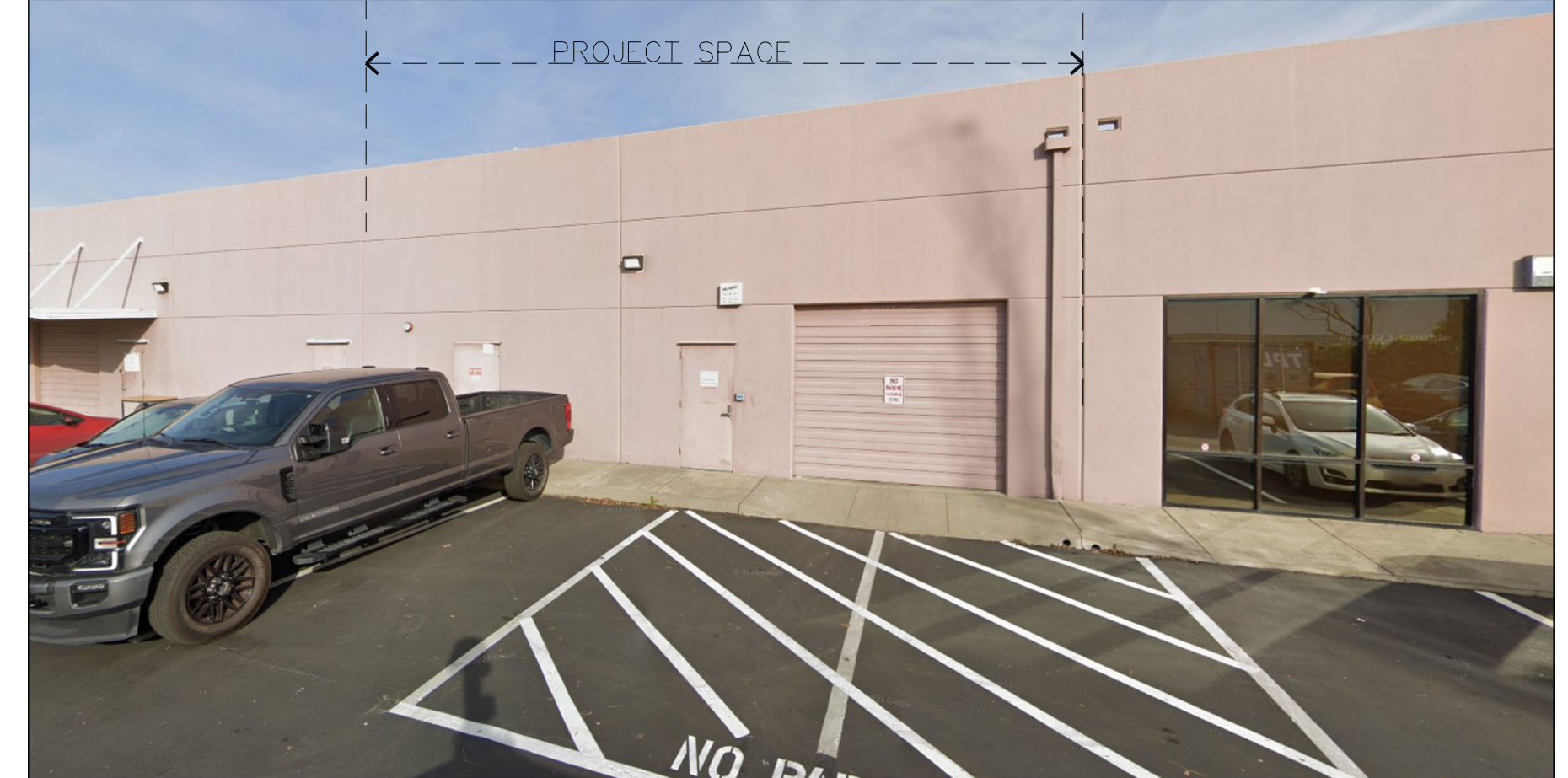
2. PHOTO OF EXISTING REAR VIEW ROLL UP DOOR TO BE REPLACED WITH WINDOW
