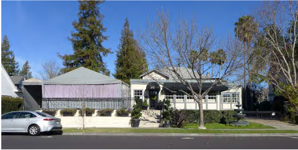
Figure 2. Looking north from St. John Street, the south façade of the main building at 475 St. John Street.
