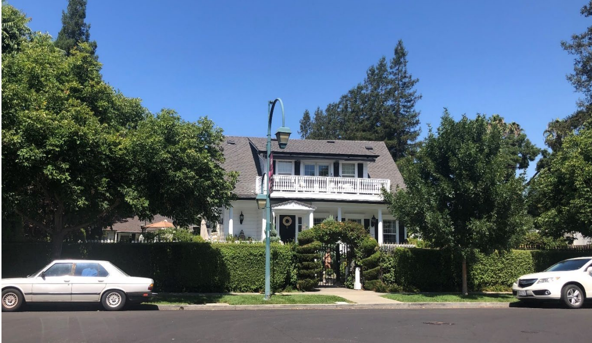
Photograph 1. Existing single-family residence at 493 St. John Street, looking north from St. John Street.
