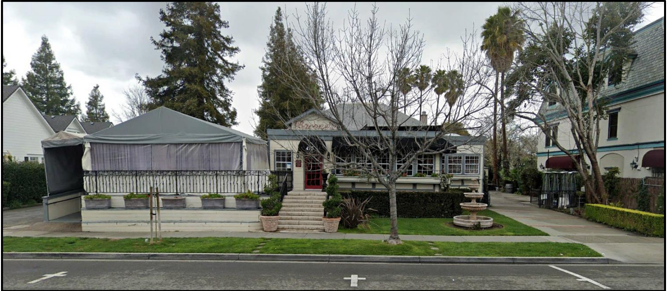
Figure 3: Street View, 475 St. John Street, Barone's Restaurant
