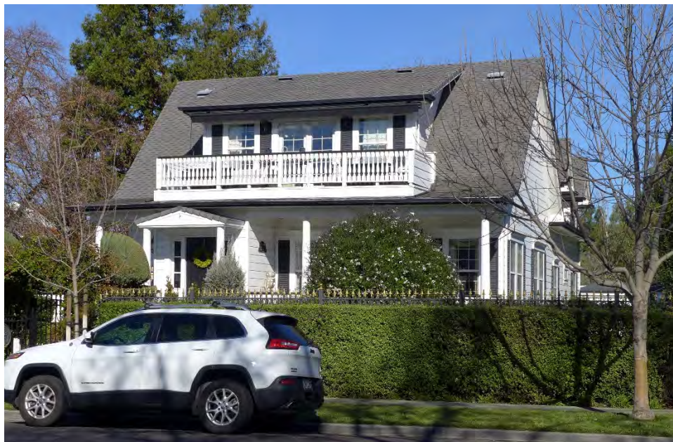
Figure 8. The front (south) façade.
