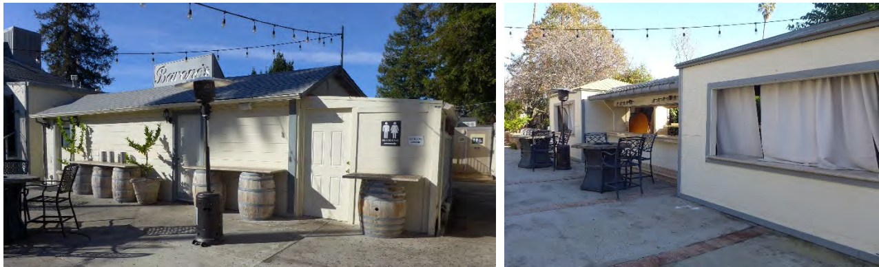
Figures 5 and 6. Two of the accessory structures on the subject parcel.
