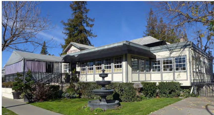
The south and east façades.
