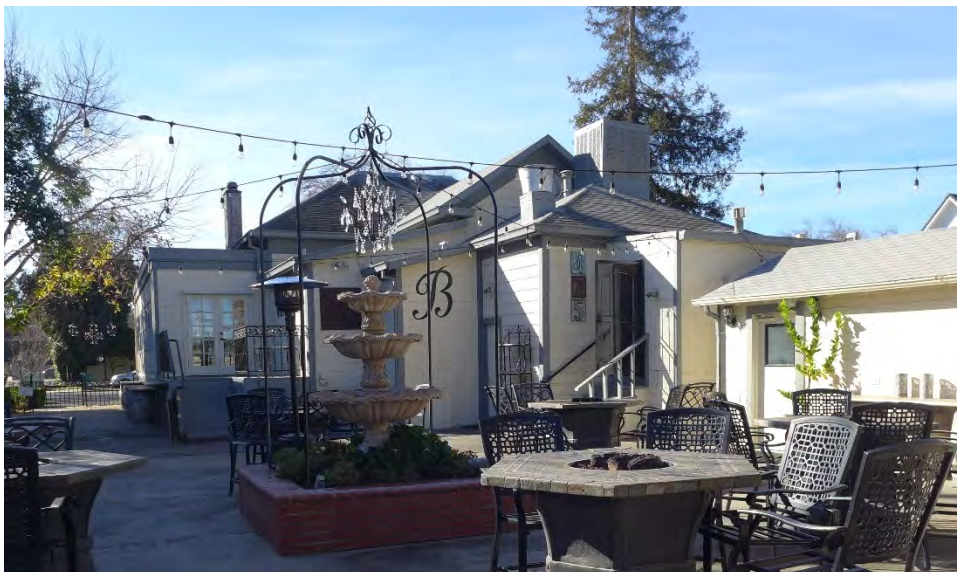
Figure 4. The rear (north) façade.
