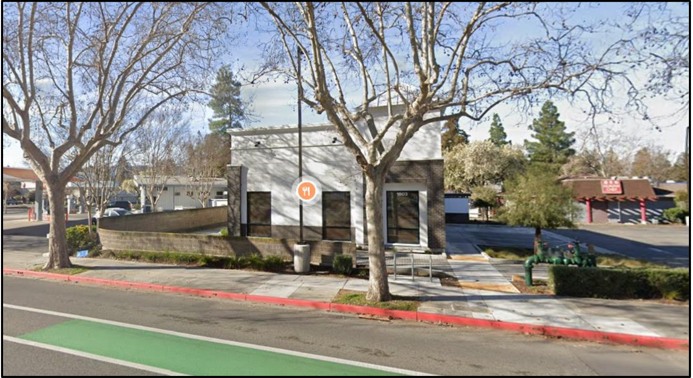
Figure 4: Current Street View of the Subject Site from Santa Rita Road
