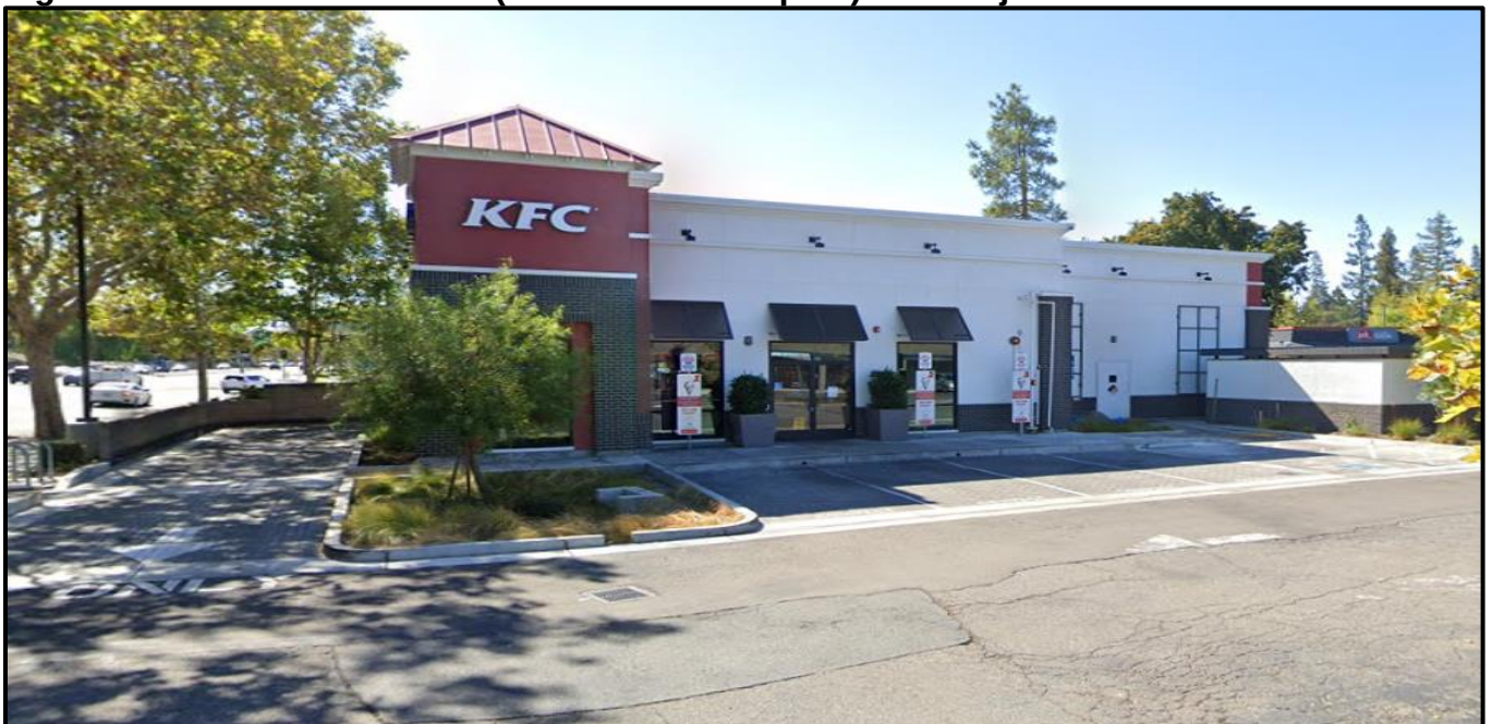
Figure 3: Internal Street View (When KFC Occupied) the Subject Site
