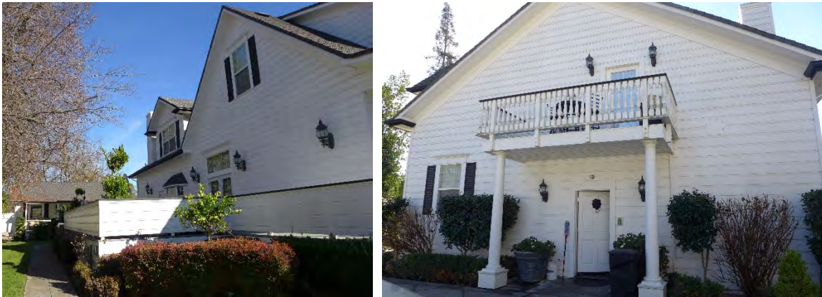
Figures 9 and 10. Left, the partial west façade, and right, the rear façade.
