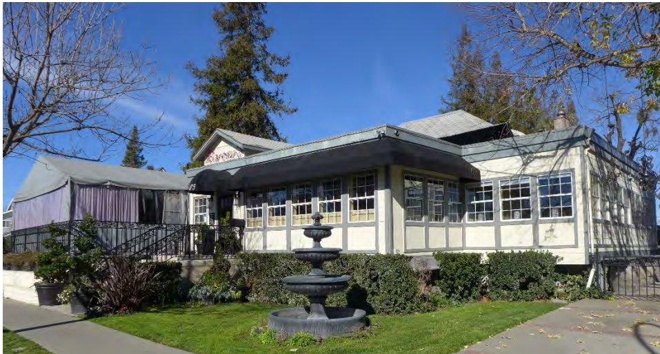
Figure 3. The south and east façades.
