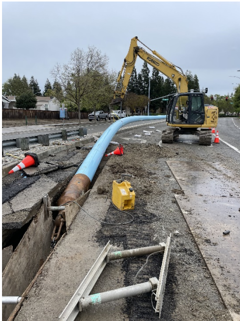
Installing water line at bridge 12" Water line in Bernal Avenue
