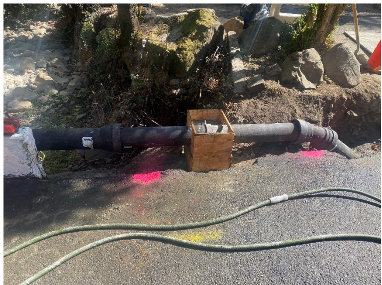
Kilkare Water Bridge Crossing
