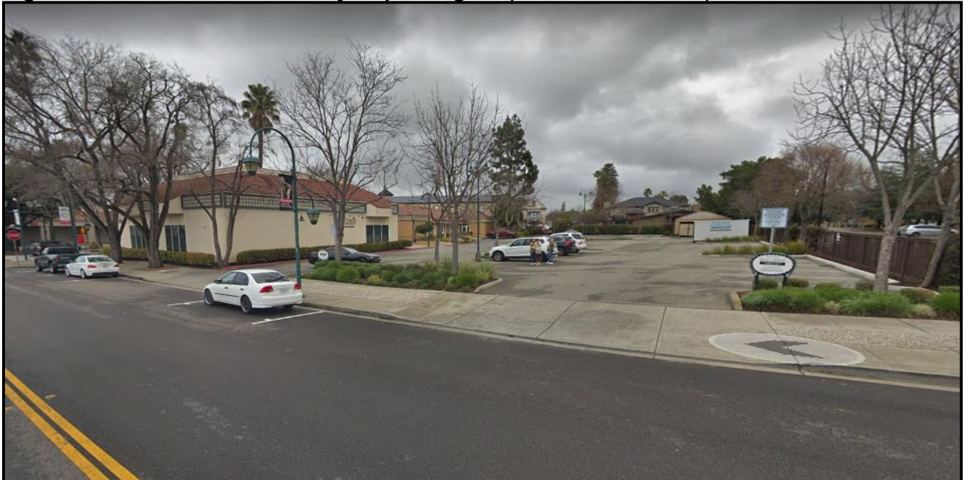
Figure 2: Street view of the subject parking lot (from Abbie Street)
