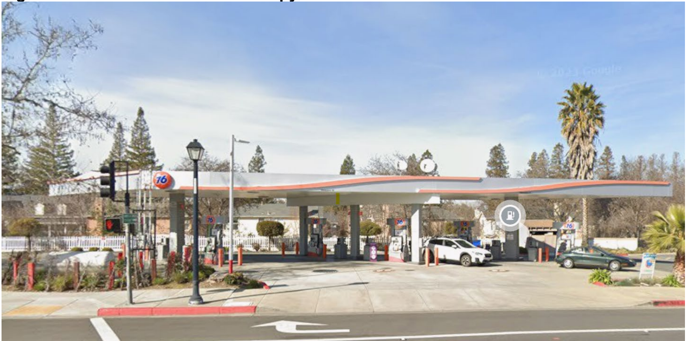
Figure 2: Previous 76 Branded canopy
